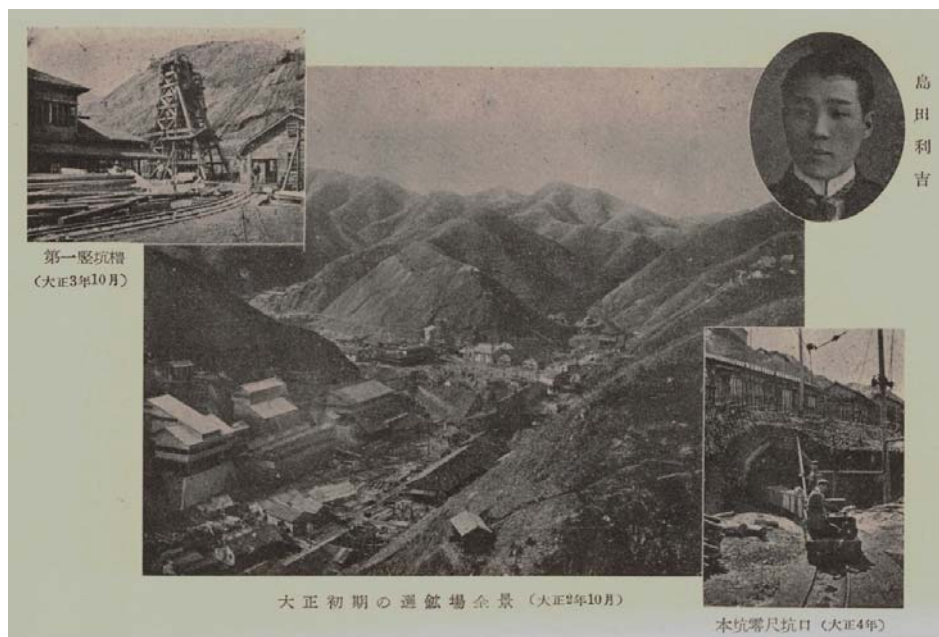
Fig.4 Distant view of Dressing Plant of Hitachi Copper Mine in early 1910's (History of Hitachi Copper Mine)
