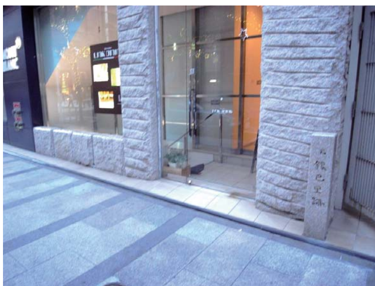
Fig.8 Re-utilization of Inada-stone (Pavement at Ginza, Tokyo Central)
